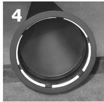
**(1). Important: A Fastite gasket must also be used, because the rubber-backed flex-ring does not perform any sealing function. 2) Placement of the flex-ring in socket and joint lubrication**
