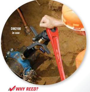
Heavy-duty Drilling Machine is compact and lightweight to make up to 2" saddle taps. Reed offers many different options to meet individual customer needs.
