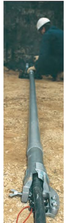
The GRUNDOMAT's reciprocating stepped-cone chisel head powers through obstructions staying on target, while conventional fixed head piercing tools are easily knocked off-course.
