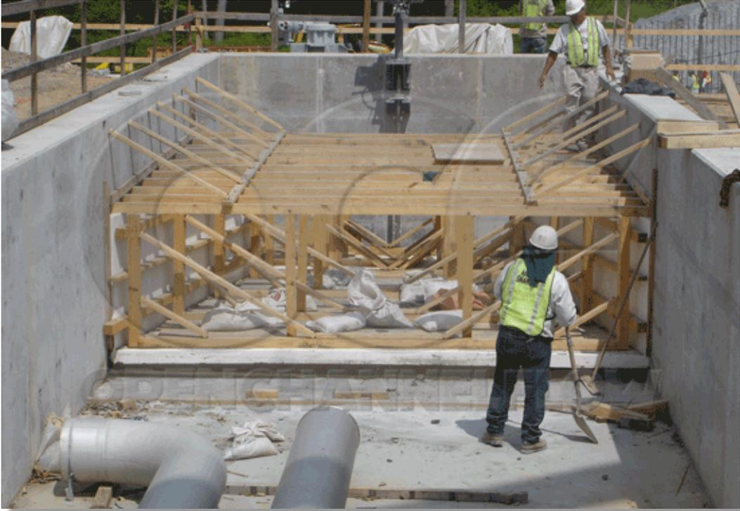
For installations where the flume is free-standing or otherwise not set in concrete, the bracing should be left in place.
