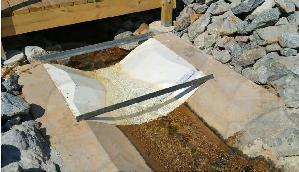
The flat bottom of the Trapezoidal flume means that it is easier to install in existing channels, passes trash quite readily, and reduces the problem of silt build-up upstream of the flume.
