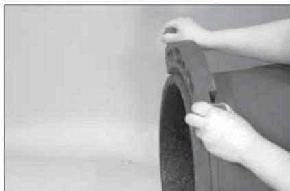
**2. ADD FIRST SEGMENT:** Place the first segment onto the pipe, making sure that the key engages in the groove properly. **NOTE:** On vertical pipe, the segments must be held in place until all segments are fastened together. For horizontal pipe, the segments can be balanced on top of the pipe, as shown above.
