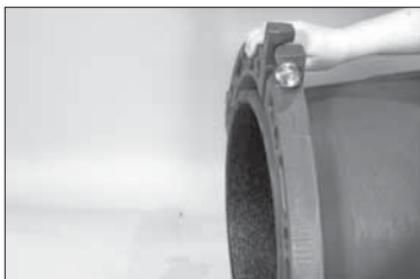
**3. ADD ADDITIONAL SEGMENTS:** Add each segment by inserting the draw bolts (provided) into the flange adapter with the nuts (provided) loosely and uniformly tightened. This will permit the flange adapter to be rotated for bolt hole alignment in later steps.
