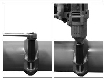
**6. TIGHTEN NUTS:** Tighten nuts evenly by alternating sides until metalto-metal contact occurs at the bolt pads. Verify that the oval neck of each bolt seats properly in the bolt hole and that housings' keys engage the grooves completely on both mating components.
