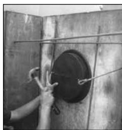
3. Place the CENTURY-LINE® Sleeve on the end cap. When field cutting non standard CS sleeve lengths, the sleeve and end caps total length should be  $\frac{1}{4}$ " longer than the thickness of the wall. Cut with a hand or power saw.
