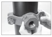
**3a.** Make sure the locating collar engages the outlet hole properly. Check this engagement by rocking the upper (outlet) housing in the hole.
