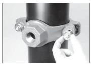
4. INSTALL REMAINING BOLT/ NUT: Insert the remaining bolt. Thread a nut onto the bolt finger-tight. NOTE: Make sure the oval neck of each bolt seats properly in the bolt hole.
