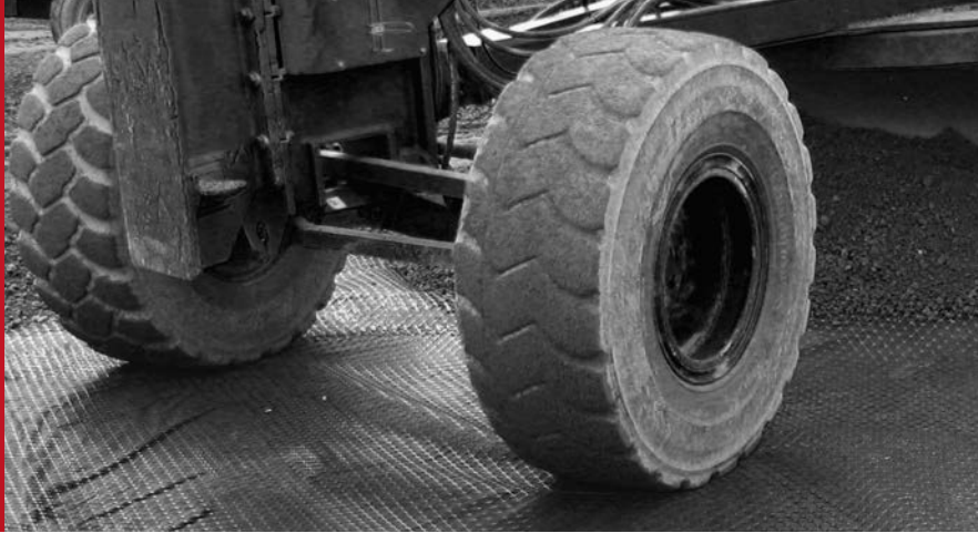
Geogrid can be trafficked directly by rubber-tired equipment.
