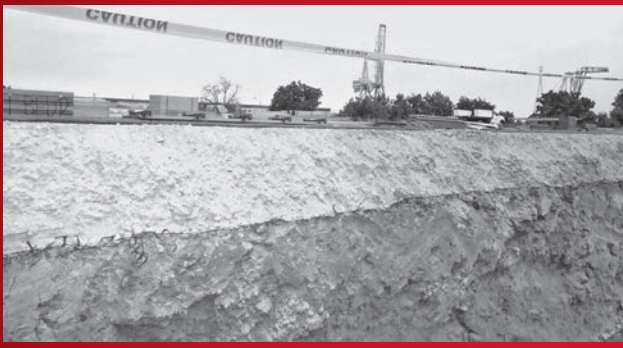
A backhoe excavation through Tensar Geogrid.
