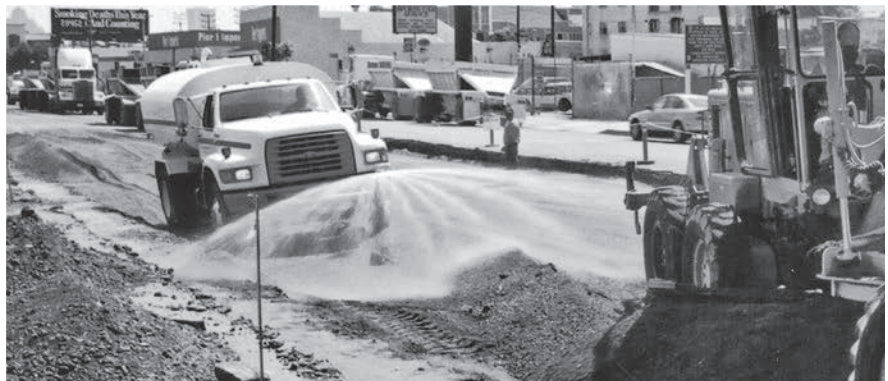
Moistening the fill before compaction.
