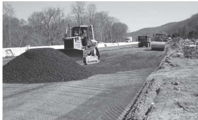
Spreading aggregate fill over Tensor Geogrid.
