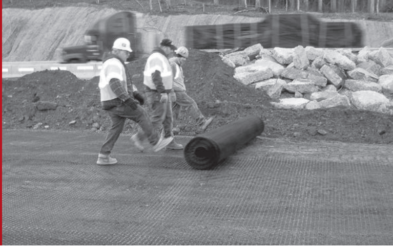
Rolling out Tensar® Geogrid.
