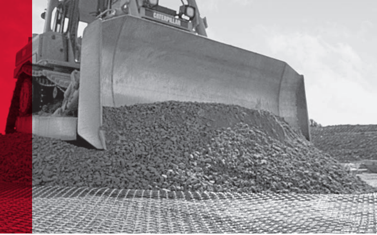
Dumping aggregate fill on top of Tensor® Geogrid over competent subgrade.
