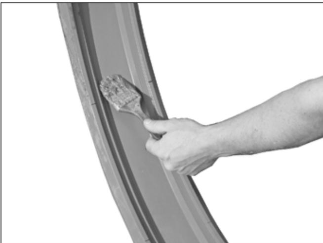
2. Check the gasket to make sure it is suitable for the intended service. The color code identifies the gasket grade. Apply a thin coat of Victaulic lubricant or silicone lubricant to the gasket lips, gasket exterior, and the interior surface of the coupling housings.
