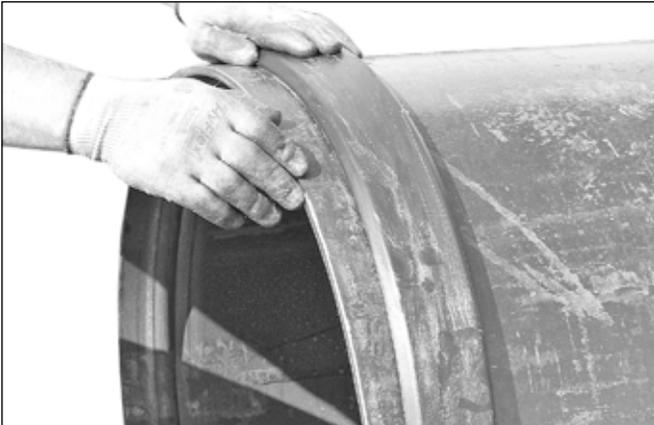
3. Position the gasket over the pipe end. Make sure the gasket does not overhang the pipe end.
