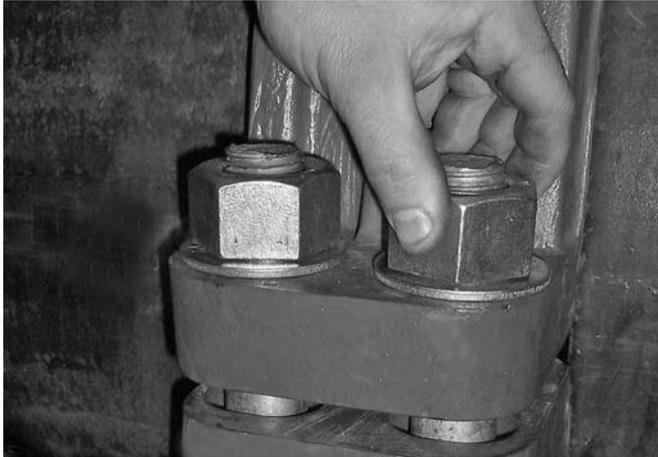
**6a.** Install a flat washer (supplied with the coupling) onto the end of each bolt, and thread a nut finger-tight onto each bolt. **NOTE:** Make sure the oval necks of the bolts seat properly in the bolt holes.
