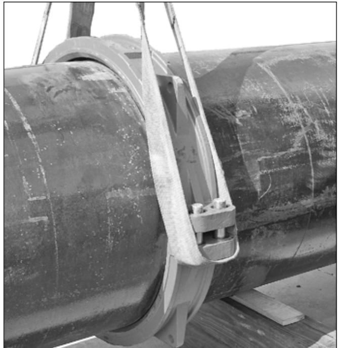
6. Using a strapping method, similar to the one shown in the photos above, install the housings over the gasket. Make sure the housings' keys engage the grooves completely on both pipes.
