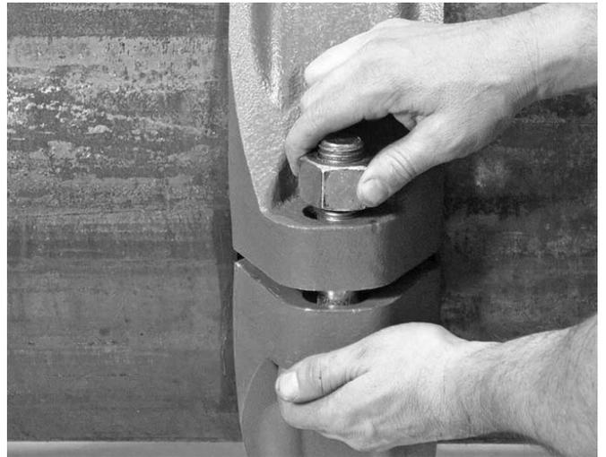
6. Install the housings over the gasket. Make sure the housings' keys engage the grooves completely on both pipes. Support the segments while preparing to install the bolts and nuts.
