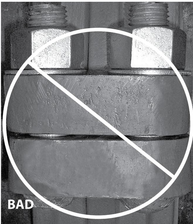
8. Visually inspect the bolt pads at each joint to ensure metal-to-metal contact is achieved across the entire bolt pad section.
