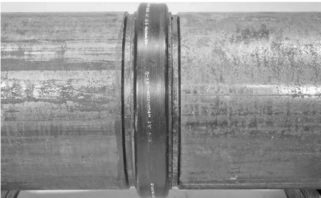
4. Align and bring the two pipe ends together. Slide the gasket into position, and center it between the grooves in each pipe.
