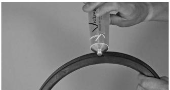
2. Check the gasket to make sure it is suitable for the intended service. The color code identifies the gasket grade. Apply a thin coat of Victaulic lubricant or silicone lubricant to the gasket lips and exterior.
