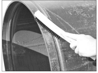
**1b.** Clean the outside surface of the pipe, from the groove to the pipe end, to remove all oil, grease, loose paint, and dirt
