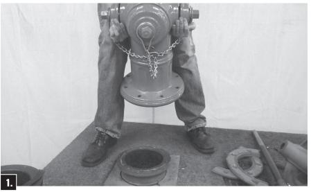
Remove stainless steel Cotter Pin from stainless steel Clevis Pin. Remove Clevis Pin and Stem Coupling from Upper Stem. Unbolt and remove broken Traffic Flange from Upper Barrel. Remove Hold-Down Nut, Anti-Friction Washer, and Operating Nut from Bonnet. Lubricate Brass Sleeve and slide over threaded Stem end to prevent O-ring damage. Unbolt Bonnet from Upper Barrel. Slide Upper Stem out of Bonnet and remove Brass Sleeve.
