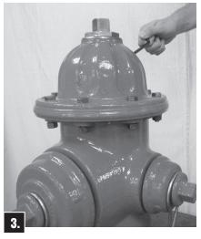
When oil is level with Oil filler Plug Hole, replace Oil Filler Plug.
