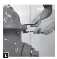
Torque Bonnet Bolts to 40-80 ft-lbs. Torque Hold-Down Nut to 200-300 ft-lbs. after Bonnet Bolts are tight. Open Gate Valve. Unscrew one Hose Nozzle Cap slightly to bleed air. Open Hydrant fully. Tighten Hose Nozzle Cap when water starts flowing and check all flange connections for leaks. Turn Operating Nut to fully closed position and remove Hose Nozzle Cap to allow Barrel to drain. Replace Hose Nozzle Cap.
