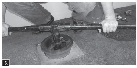
Tighten Main Valve to 100-150 ft-lbs. Turn on water at the Gate Valve and remove Wrench from Stem by removing Clevis Pin.
