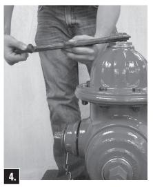
Tighten Operating Nut, turning in closing direction.
