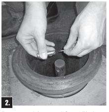
Remove stainless steel Cotter Pin from stainless steel Clevis Pin in Lower Stem (throw away the old Clevis Pin, Cotter Pin, and old coupling).
