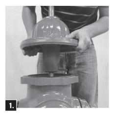
Remove Hold-Down Nut Operating Nut and Anti-Friction Washer from Bonnet. Lubricate Brass Sleeve and slide over threaded stem to prevent O-ring damage. Unbolt and remove Bonnet. Remove Brass Sleeve.
