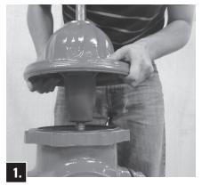
Remove Hold-Down Nut, Anti-Friction Washer and Operating Nut from Bonnet. Lubricate Brass Sleeve and slide over threaded stem end to prevent O-ring damage.
