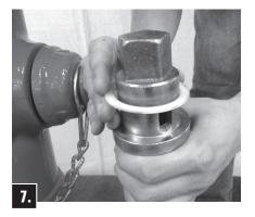
Check Bonnet O-ring\* for proper position and condition. Attach Brass Sleeve to Upper Stem and lubricate outside to protect O-ring Seals from thread damage. Place Bonnet onto Upper Barrel and assemble Bonnet Bolts only hand-tight. Remove Brass Sleeve. Reassemble Operating Nut, Anti-Friction Washer, and Hold-Down Nut (snug-tighten). Be sure O-ring Seals are in good condition at thread shoulder on outside of Hold-Down Nut and on inside where contact is made with Operating Nut.
