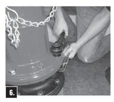
Reassemble Upper Stem to Lower Stem. Place Upper Barrel in place and reassemble Traffic Flange.\* Tighten Bolts to 60 ft-lbs.
