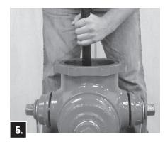
Lower Main Valve into the Barrel.
