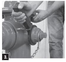
Place Nozzle Wrench, A-316, on Nozzle with Wrench Forks facing toward Hydrant Barrel and locked onto Nozzle Drive Lugs. Replace Nozzle Cap and tighten until Cap rests loosely against backside of Wrench. Remove Nozzle (nozzle threads out in a clockwise rotation). Additional leverage may be obtained by placing a length of 2" schedule 40 steel pipe over the handle of the Nozzle Wrench.
