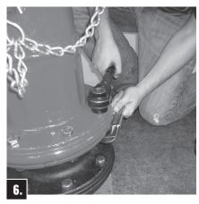
Attach Upper Barrel with Traffic Flange Halves (with bevel on outer edge downward) and Bolts; being sure Traffic Flange O-ring\* is in groove in Upper Barrel. Tighten Bolts to 60 ft-lbs.
