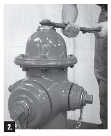
Turn Operating Nut slightly in the opening direction to relieve compression between Barrel sections.
