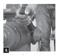
Install Nozzle O-ring on the inlet side of the Nozzle. Thread new Nozzle into Upper Barrel, attach A-316 Nozzle Wrench as described in Step 3, and tighten Nozzle (nozzle threads in a clockwise rotation) to approximately 600 ft-lbs torque (100 lbs. pull on a 6' lever).
