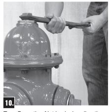
Turn Operating Nut in closing direction to make sure Main Valve is closed tightly, then turn in opening direction approximately 1/4 turn to relieve tension on operating mechanism.
