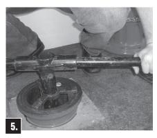
Tighten Main Valve to 100-150 ft-lbs. Turn on water at the Gate Valve and remove Wrench from Stem by removing Clevis Pin.
