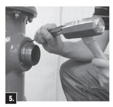
Remove Nozzle Cap and A-316 Nozzle Wrench. Place the Nozzle Lock (Part 143137), lengthwise in the slot formed by the Nozzle Drive Lugs and the Barrel Bore. Drive the Nozzle Lock in place by striking the Nozzle Lock Installation Tool (Part 143132) several times with a heavy brass hammer.
