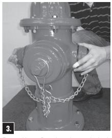
Rotate Upper Barrel section as desired.
