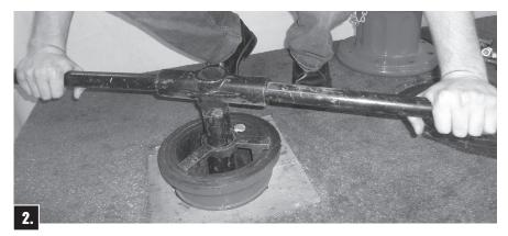
Slide slotted end of Wrench over Lower Stem. Align holes in Wrench and Stem and attach Wrench to Stem with Clevis Pin. Lower Support Arm onto the Flange of Lower Barrel and tighten Thumb Screw (to hold Main Valve in closed position). Remove Main Valve Assembly by turning Wrench counter-clockwise and lift out Wrench, Lower Stem, Main Valve Assembly and Seat Ring from Hydrant Barrel as a unit.
