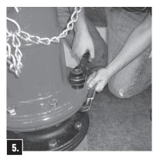
Attach Upper Barrel with new Traffic Flange Halves (with bevel on outer edge downward) and Bolts; being sure Traffic Flange O-ring\* is in groove in Upper Barrel. Tighten Bolts to 60 ft-lbs.
