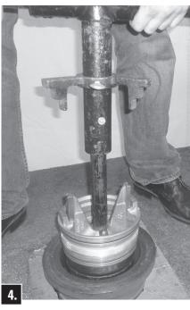
Lower Main Valve into the Barrel. Lower Support Arm and tighten Thumb Screw. Carefully thread main valve assembly clockwise into the base of the Hydrant. Hand tighten.
