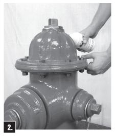
If oil is low, use a small funnel to add MUELLER Hydrant Lubricant.
