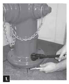
Loosen Nuts on Traffic Flange Bolts.
