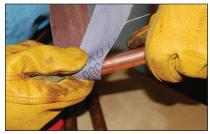
Clean all copper pipes and fittings with Oatey high carbon steel brush, abrasive cloth, emery cloth or other abrasive materials, then wipe with a clean cloth.
