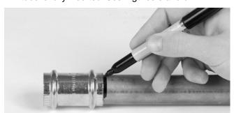
Figure 8 - Marking the Tubing After Fully Inserting Tube
