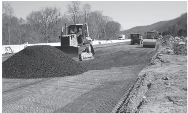
Spreading aggregate fill over Tensor Geogrid.
