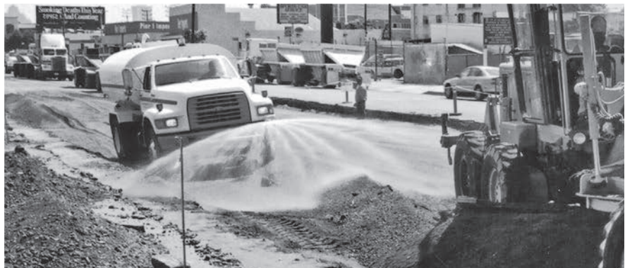
Moistening the fill before compaction.
