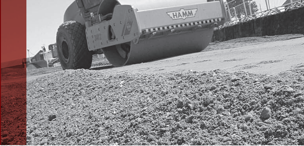
Compacting the aggregate fill.
