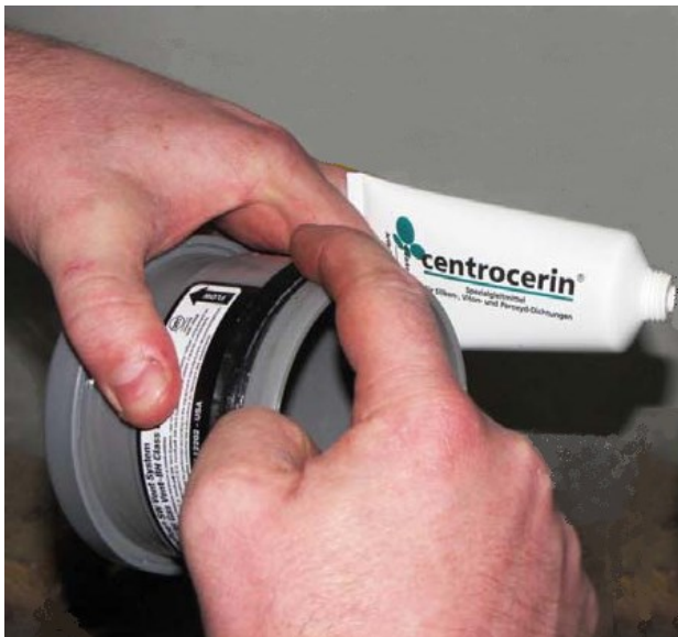
Figure 5: Applying Lubricant to Gasket
