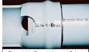
Photo # 11: Properly Inserted Spigot
