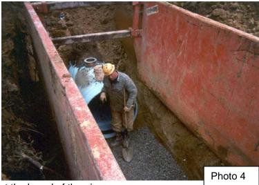
to reduce axial deflection and support the barrel of the pipe.
