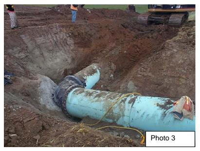
Foundation: An adequate or stable foundation should be present (or provided) to uniformly support the full length of the pipe. Bell holes should be provided at each joint to permit proper assembly and support of the pipe. Unstable trench bottoms shall be stabilized by methods and with materials required, by the specifying engineer, to provide adequate and permanent support for the conditions encountered.
