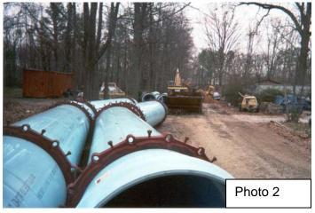
installed in the haunching area. Refer to Figure 1 for the location of the haunch area. Where embedment compaction is required, the trench shall be wide enough to accommodate the compaction equipment. If minimum trench width is exceeded, and embedment compaction is required, pipe zone haunching should be compacted at least one pipe diameter from the pipe on both sides of the pipe.
