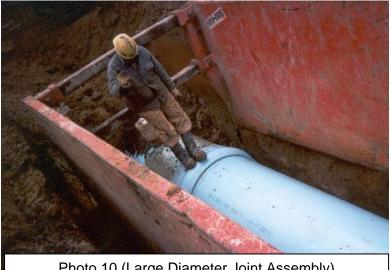
Photo 10 (Large Diameter Joint Assembly)
