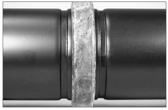
**3. JOIN MATING COMPONENTS:** Align the two grooved mating component ends. Insert the other mating component end into the gasket until it contacts the center leg of the gasket. **NOTE:** Verify that no portion of the gasket extends into the groove of either mating component
