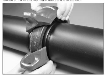
**7. INSTALL HOUSINGS:** Install the housings over the gasket. Make sure the housings' keys engage the grooves properly on both pipes/mating components.
