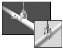
**Note:** Threaded rod shall not come in contact with CPVC when installed. It is advisable to use lift restraint devices such as those produced by Tolco and Afcon that prevent the threaded rod from coming in contact with the CPVC pipe (as shown above).
