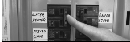
Figure 27 - Circuit Breaker
