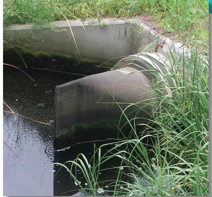
Detail of the *ProFlex*<sup>TM</sup> Slip-on Rubber Check Valve; Style 730
