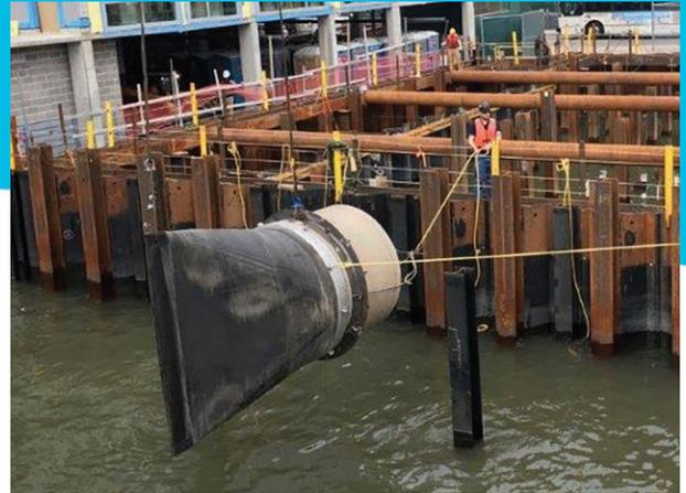
Detail of the *ProFlex™* Flanged/Slip-On Slope Bottom Check Valve; Style 731
