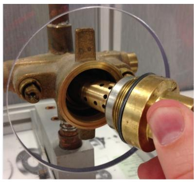
3) Notice how the TA-10 spindle rests up against the T-12A cap. This is assurance that the valve was open fully to the hot water position before trying to remove the cap. *Failure to do so can damage the cap and spindle and make it extremely difficult to remove the spindle from the valve.* Rotating the spindle counter clockwise, remove the spindle from the cap assembly.
