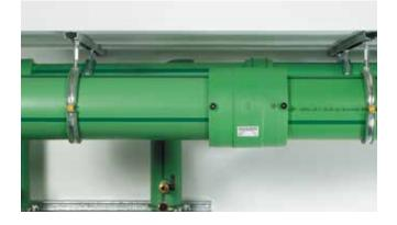
9. Make sure the pipes are free from bending or the stress of their own weight within the Aquatherm electrofusion socket. The socket should be movable at both pipe ends after assembling. The air gap must be even around the circumference. A stressed or displaced connection can cause an unacceptable melt flow and a defective connection while joining. The pipe ends and electrofusion socket must be dry during installation.
