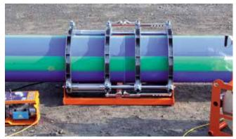
Join the pipes and cool under pressure.
