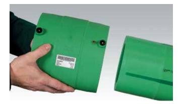
8. Push the other prepared pipe end into the Aquatherm electrofusion socket. Tighten the clamps (if using any).
