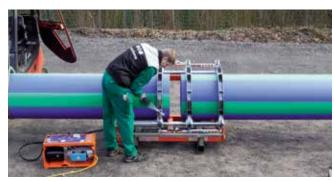
The parts to be welded are fixed.
