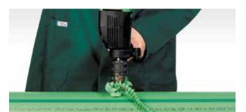
Drilling through the pipe wall.
