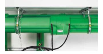
14. Do not move or stress pipe and fitting during the fusion process and cooling time. The fused pipe joint must not be moved (no release of the clamps) or stressed before complete cooling. The minimum required cooling time is marked on each Aquatherm electrofusion socket. Ambient temperatures of more than 77 °F (25 °C) or connections in direct sunlight need longer cooling times. The Aquatherm electrofusion sockets are rated up to 300 psi.
