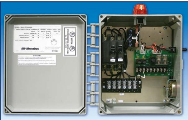
This single phase simplex control panel, designed for and **accepted by the Wake County Regulators**, provides an effective, reliable means of controlling one single phase pump in water and sewage installations. **Also approved for Burke, New Hanover and Pender counties.**
