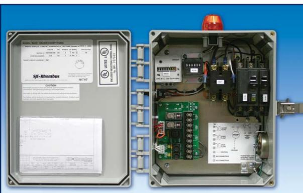
This single phase simplex control panel, designed for and **accepted by Wake and Orange County Regulators**, provides an effective, reliable means of controlling one single phase pump in water and sewage installations. **Also approved for Craven county.**
