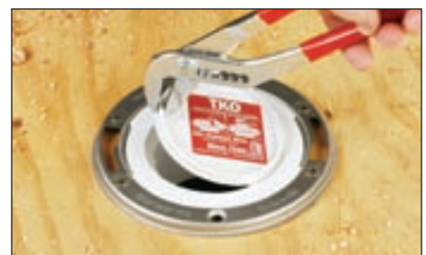
Remove loose knockout with pliers.
