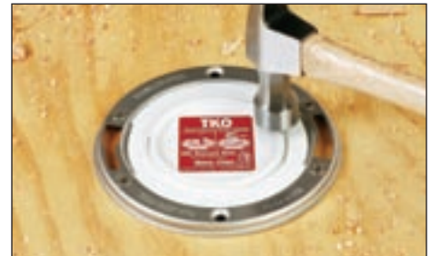
Hit the raised rim of the TKO until the knockout cracks loose.
