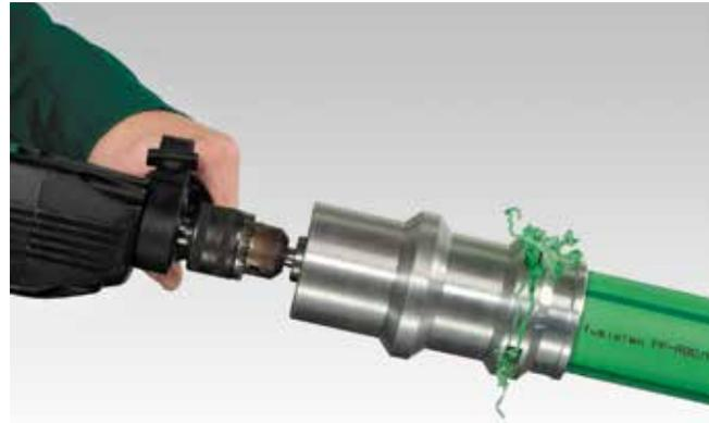
5. Clean the pipe again thoroughly, removing any burrs and smoothing the surface of the pipe.
