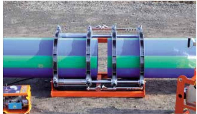
Open the clamps and remove heating element.
