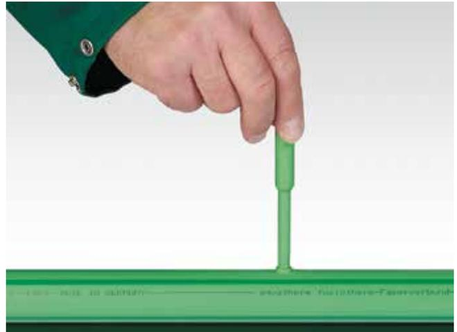
7. Cut away the unused portion of the repair pin. Wait at least two minutes before turning the system back on.
