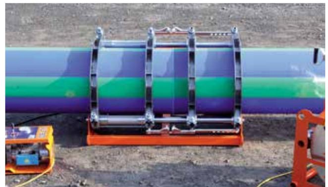
Join the pipes and cool under pressure.
