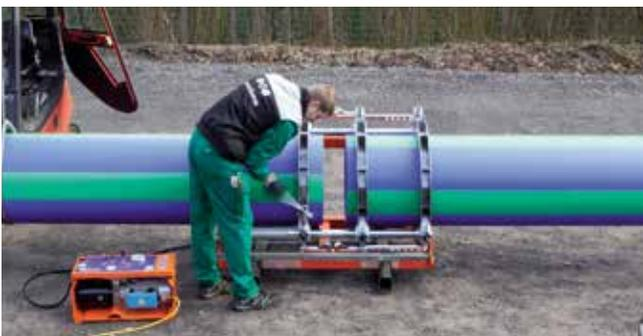
The parts to be welded are fixed.
