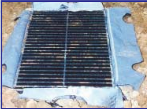
installed Siltsack held in place by grate.
