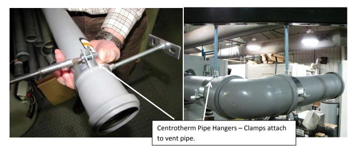
Steel joint connector rings (available from Centrotherm supplier) must be used at each pipe joint. The connector rings ensure that the joints do not separate under heavy loads. These connector rings must be used to comply with ULC-S636 requirements. See following photo with the joint connector attached to the pipe sections.
