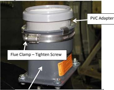
Commercial Power Direct Vent Exhaust Outlet Adapter
