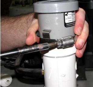
For the exhaust venting for all power vent and power direct vent models, insert the PVC Adapter into the Exhaust Outlet Adapter. On residential models, tighten the clamp to secure the PVC Adapter.
