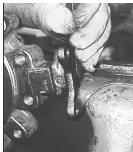
Figure 4 – Shows how the upper stem is removed from the upper disk hub.
