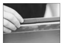
Apply Neoprene gasket completely around WDCI frame to the beginning point. Butt the two ends of the gasket up against each other. Do not overlap the two ends.
