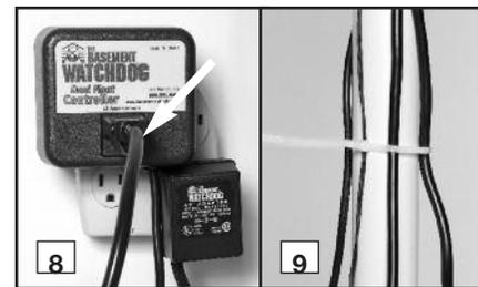
9. For a neater installation, secure the cables from the controllers to the discharge pipe in a couple places with the additional cable ties. Make sure the wires are not touching each other or overlapping each other.
