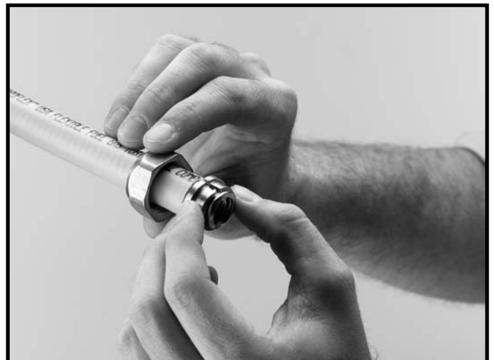
Step 2 Slide nut over tubing and place retainer ring. Leave one corrugation exposed on the end of tubing.
