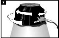
Using a moderate to high flame, begin heating the sleeve from the bottom edge. Apply heat circumferentially around the structure. Continue heating upward as the sleeve shrinks. Use a gloved hand or roller to smooth wrinkles and push out trapped air.
