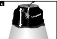
Place the closure seal on a flat surface (adhesive side up) and apply gentle heat to activate the adhesive. Center the closure vertically over the overlap and apply a small amount of heat to the face of the closure. Using a gloved hand pat the closure down and, alternating with heat and pressure. Continue until the closure is fully bonded.
