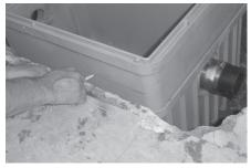
Locate the assembly on to the tank insuring that it is fully seated between the location points. Determine if the extension assembly needs to be shortened and mark accordingly.
