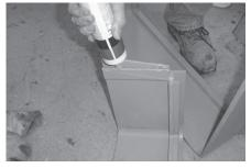
Apply a generous bead of silicone to the tongue and groove channel on the ends of the extension components.
