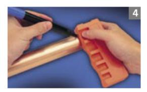
5) Insert the tube fully into the fitting until it meets the tube stop. With the fitting in place, clearly mark the tube outside diameter at the edge of the fitting. As an alternate, an XPress depth gage may be used to properly locate the insertion depth as shown in photograph 4.
