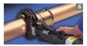
6) Press the trigger or the actuation button on the pressing tool and complete the pressing operation. Please refer to the tool manufacture's instructions for more detail. Inspect the pressed joint to ensure the tube has remained fully inserted during the pressing operation.
