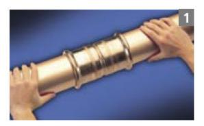
1) Assemble the joint, ensuring that the tube is inserted into the fitting until it meets the tube stop. Check the insertion depth by using the mark placed on the tube outside diameter during step 4 of preparation. The pressing operation should only be undertaken with the tube fully inserted into the XPress fitting.
