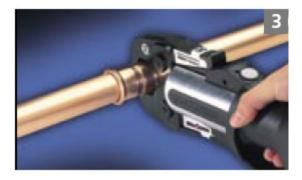
3) Depress the pressing tool trigger or actuation button to begin the pressing cycle. The cycle is complete when the jaw fully encloses the mouth of the fitting. The jaw should then be released from around the fitting. Please refer to the tool manufacture's instructions for more detail. Inspect the pressed joint to ensure the tube has remained fully inserted during the pressing operation.
