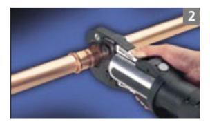
2) With the correct size pressing jaw inserted into the pressing tool, place the jaw over the bead on the fitting. Great care should be taken to ensure that the pressing tool and jaw are maintained at a  $90^{\circ}$  angle to the tube centerline.
