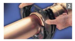
2) Select the appropriate size pressing ring, open it by depressing the spring loaded pin (check manufacturer's operating instructions). Open the pressing ring jaws and position it over the fitting.
