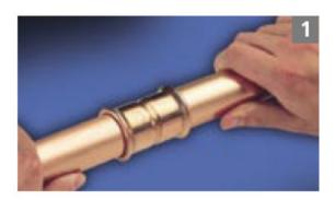
1) Assemble the joint, inserting the tube into the fitting until it meets the tube stop. Check the tube insertion depth using the reference mark on the tube outside diameter, see step 4 in the preparation process. The pressing operation should only be undertaken with the tube fully inserted into the XPress fitting. Note – Clean water may be used to ease the assembly process. Wetting the tube and or the fitting will ease the tube insertion process.
