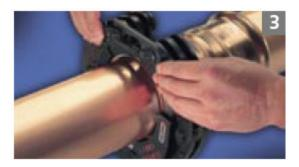
3) Align the groove in the pressing ring with the bead on the outside diameter of the XPress fitting. Fit the support plate on the pressing ring over the tube side of the joint as shown.
