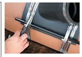
7. Tighten clamps to 60 inch-lbs. torque. Test for leaks prior to backfilling.
