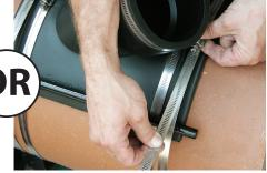
**NOTE:** For TSW-4 ONLY Due to space restrictions, install the 2 clamps provided around the host pipe **OUTSIDE** of the tap saddle bands.
