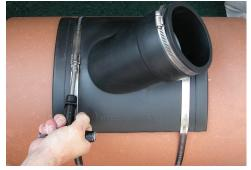
**3.** Install the appropriate Fernco Flexible Tap Saddle as needed. Tighten clamps to 60 inch-lbs. torque.
