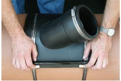
**4.** Attach the reinforcing bars to the saddle by sliding the clips under the saddle.
