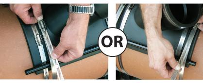
6. Install the 2 clamps provided around the host pipe near the saddle inlet, **INSIDE** of the tap saddle bands.
