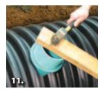
Using a hammer and block of wood, drive the pipe stub to the QwikSeal pipe stop.
