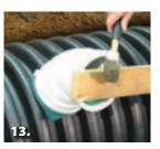
Install pipe fitting. Fitting should sit flush with the surface of the QwikSeal.
