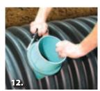
Install the band clamp at 60 in-lbs. torque.
