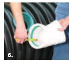
Measure the depth of the fitting to be attached to the pipe stub. See alternative method below.
