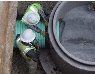
For rubber boot connection two "flat top" gaskets are positioned under the boot to ensure a water tight seal. Manhole boots should be sized to fit the outside diameter of CORR-21.
