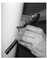
Figure 9.1: Drill and Tap Combustion Test Port
