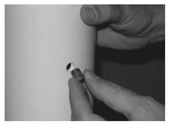
Figure 9.3: Insert Pipe Plug into Test Port
