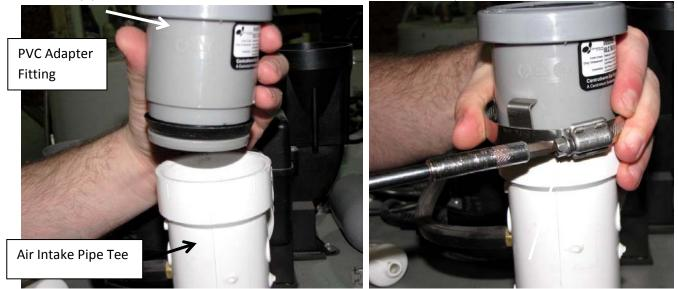
For the exhaust venting for all power vent and power direct vent models, insert the PVC Adapter into the Exhaust Outlet Adapter. On residential models, tighten the clamp to secure the PVC Adapter. For Commercial Power Direct Vent models, insert PVC Adapter into Exhaust Outlet Adapter. Install Flue Clamp over Exhaust Outlet Adapter and Tighten clamp screw to secure the PVC Adapter.
