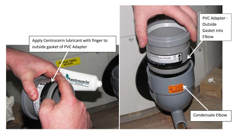
Install Centrotherm Flue Clamp around outside of elbow so that Clamp Brackets engage PVC Adapter shoulder as shown. Tighten Flue Clamp Screw to secure PVC Adapter into Condensate Elbow
