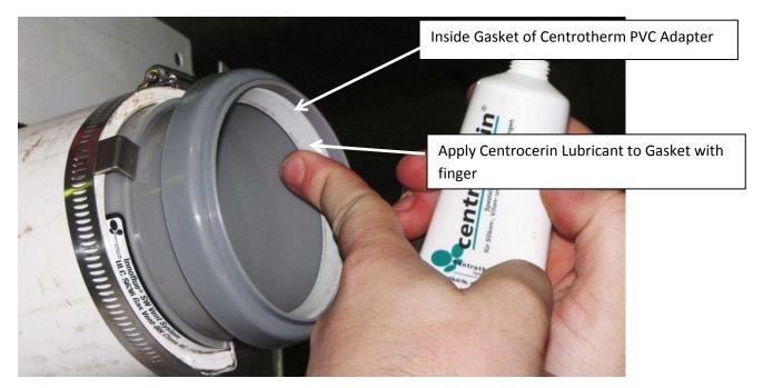
Insert the male end of the straight pipe or elbow into the flanged gasketed end of the PVC adapter. Push the pipe or elbow into the adapter using a twisting motion to fully insert the pipe into the gasket inside the adapter.
