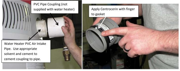
Insert male gasketed end of Centrotherm PVC adapter into PVC pipe coupling.
