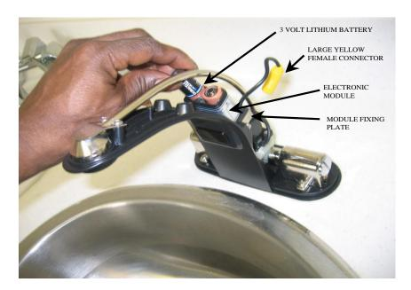
5b. When installing the AC powered version **(S-9020)**, connect the AC cable assembly to the cable attached to the transformer **(Black connectors)** and plug the Transformer into a standard 120 VAC outlet. The AC operated electronic module is now ready to activate the unit. Attach AC cable to wall with the wire clip provided for a more secure installation. The transformer can be located behind the wall out of the reach of vandals. Multi-unit transformers are also available, see Section IV.
