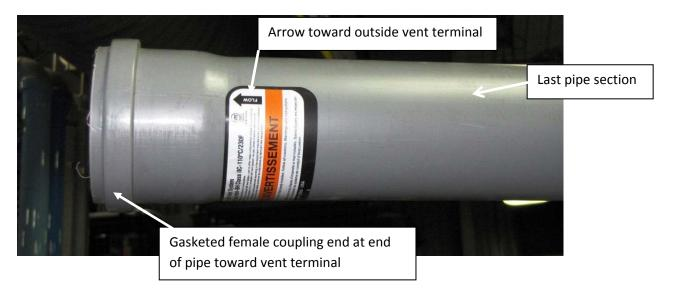
Install the appropriate diameter Centrotherm ISTAGL PVC Termination Adapter on the end of the last pipe.
