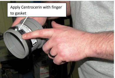
Insert male gasketed end of Centrotherm PVC adapter into PVC pipe coupling.
