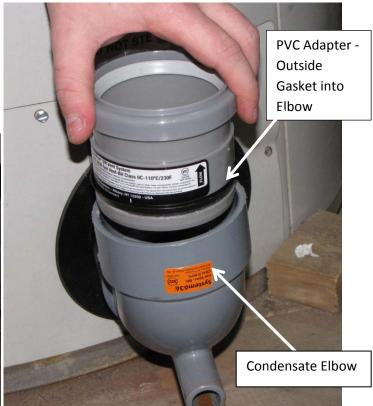
Install Centrotherm Flue Clamp around outside of elbow so that Clamp Brackets engage PVC Adapter shoulder as shown.
