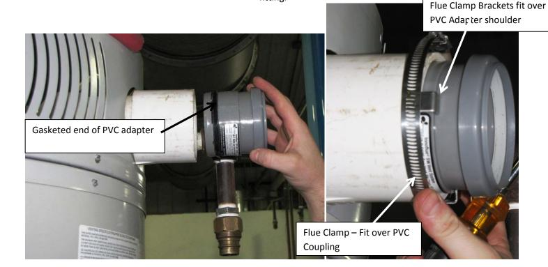
Tighten clamp screw securely to secure the PVC Adapter to the cemented PVC coupling. Refer to the instruction manual for appropriate solvent and cement.
