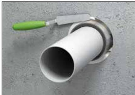
5. Fill the gap with fire-resistant acrylic, foam or mortar
