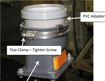
Commercial Power Direct Vent Exhaust Outlet Adapter
