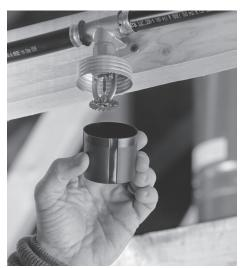
Keep heads within protective shell during installation
