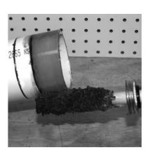
Apply a second coat of primer to the fitting socket aggressively working it into the surface.
