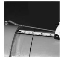
• To ensure joint integrity, once insertion is complete, the pulling tool can be used to hold the joint in place during set time and also to ensure that the pipe does not back out.
