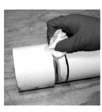
• Align all piping system components properly without strain. Do not bend or pull pipe into position after being solvent welded.
