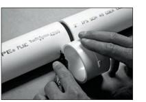
Place the repair coupling on the pipe with the larger pipe ID (inside diameter) end facing the gap between the pipe ends.
