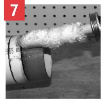
yond the hub depth. Aggressively work the cement into the surface.
