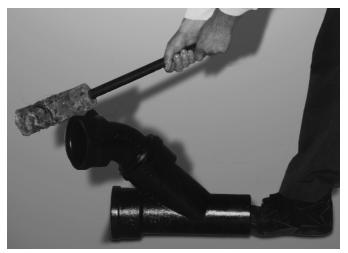
• **Using a Lead Maul.** Almost all plain-end fittings may be installed by driving them into place with a lead maul or a mallet. After installing and lubricating the gasket, align the spigot and strike the fitting on its driving lug, or across its full hub, with a lead maul. Driving lugs are standard on all Charlotte plain-end bends and they make joining easy. The fitting may be struck as hard as necessary, since the lead maul will deform before damaging the fitting.
