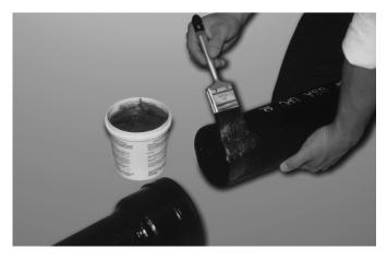
For large-diameter pipe and fittings (5" - 15"), we recommend that you use an adhesive lubricant.
