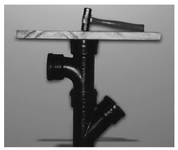
• **Using a Mallet.** If you prefer to use a mallet, place a wooden block over the fitting's hub. After installing and lubricating the gasket, align the spigot and strike the wooden block with the mallet until the spigot is properly seated.
