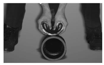
• **Double Folding:** Squeeze the gasket together with both hands, then insert it into the hub. As you withdraw your hands, the gasket will unfold, or snap into proper position.
