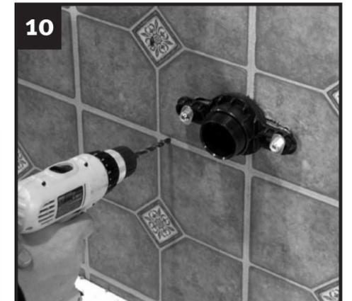
10 Drill holes for the lower anchor screws.
